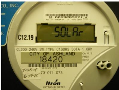
**Screen 4:** This screen is just to show that the meter is programmed for a solar installation. It is only a convenience screen so that meter readers and installers know that it is reading both directions.
