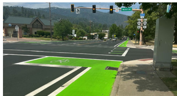
Pictured above is the new bike box at the intersection of Ashland St and Walker Ave. Drivers are not permitted to make a right turn at a red light where bike boxes are present.
